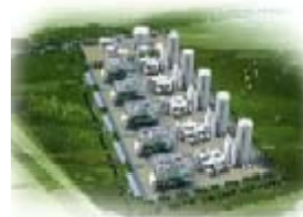
Air Separation Plant Site
